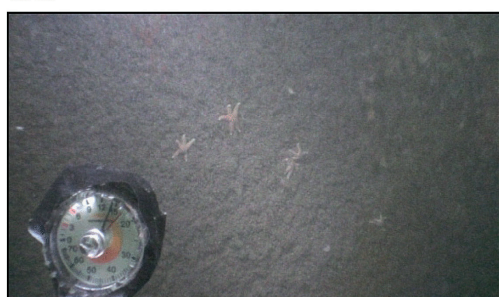
Figure 3. Growth in the subtidal zone of a monopile in owez. Video stills collected by Wals Diving, figure by Bureau Waardenburg.
