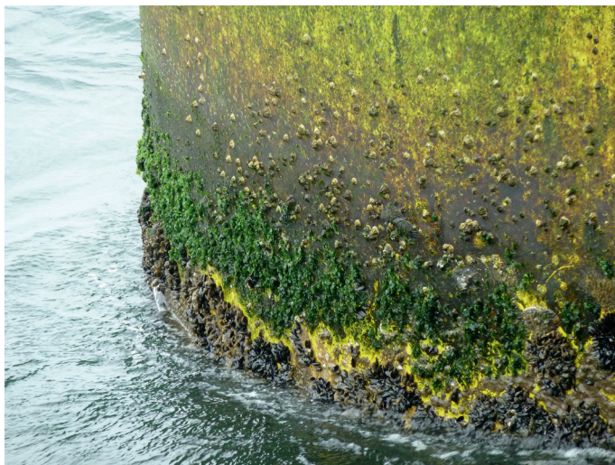
Figure 2. Growth in the intertidal zone of a monopile in OWEZ. Photo Sietse Bouma.
