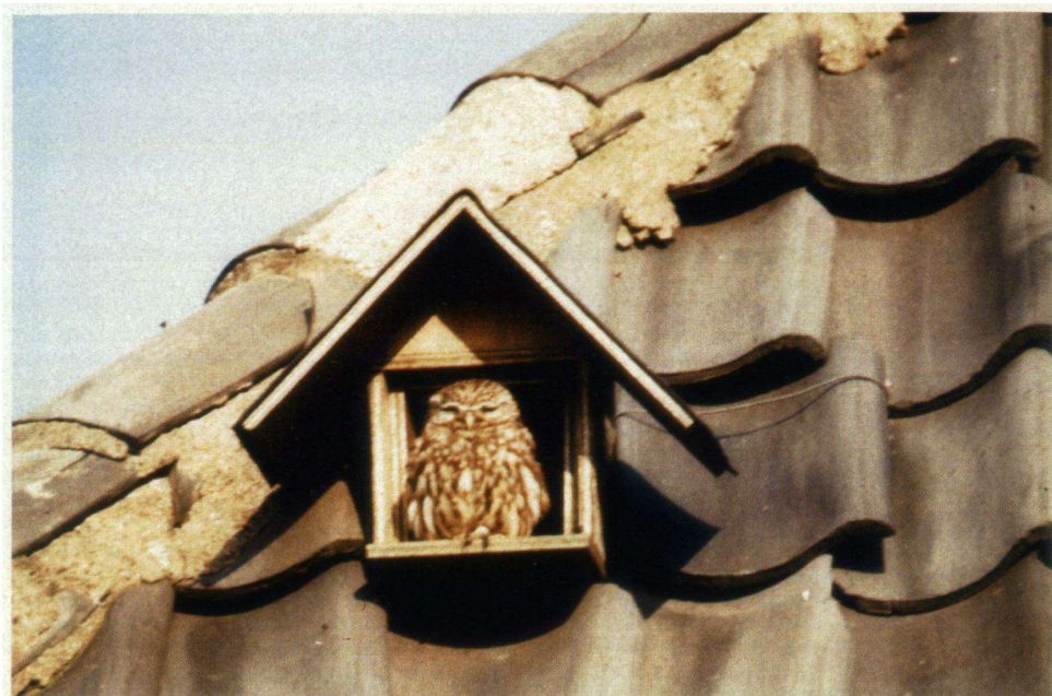
Steenuil op 'balcon' ten behoeve van 'Day by day' monitoring.
